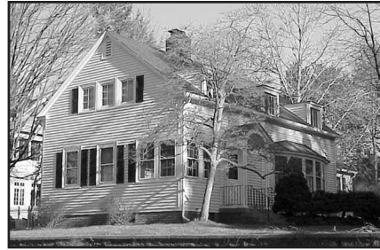
George Grennell House, pre-1846 53 High Street. Private Residence.
