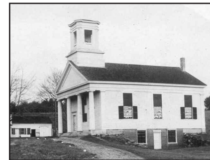
Coldbrook Springs Baptist Church, original location Image courtesy Peter S. Miller
